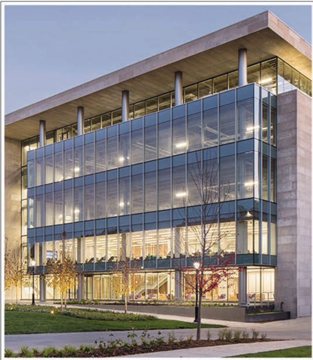
The Northwestern University Mudd Hall Expansion Project was 100% BIM coordinated and took full advantage of Block Electric's new fabrication shop run by Luke Simpson.
