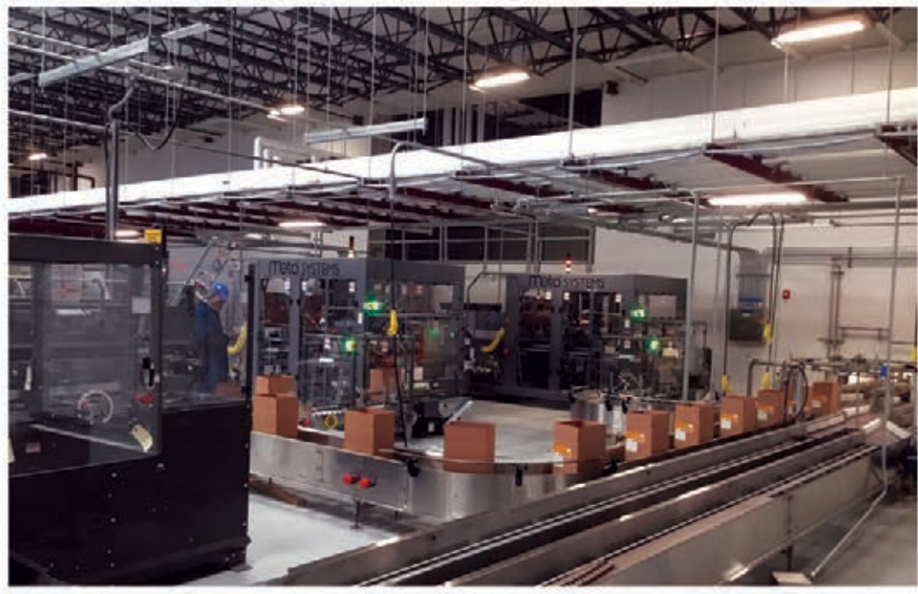
The Costco Meat Plant in Morris, Illinois is very close to completion and already producing hot dogs. This 281,000 square foot production facility will greatly improve deliveries to the Midwest and East coast. (See story on page 3)
