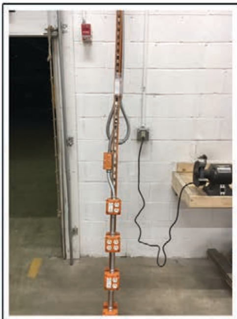
Free-Standing Temp Power Poles
