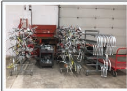
Pre-Bent Stub-Ups & Boxes with Brackets on Mobile Carts
