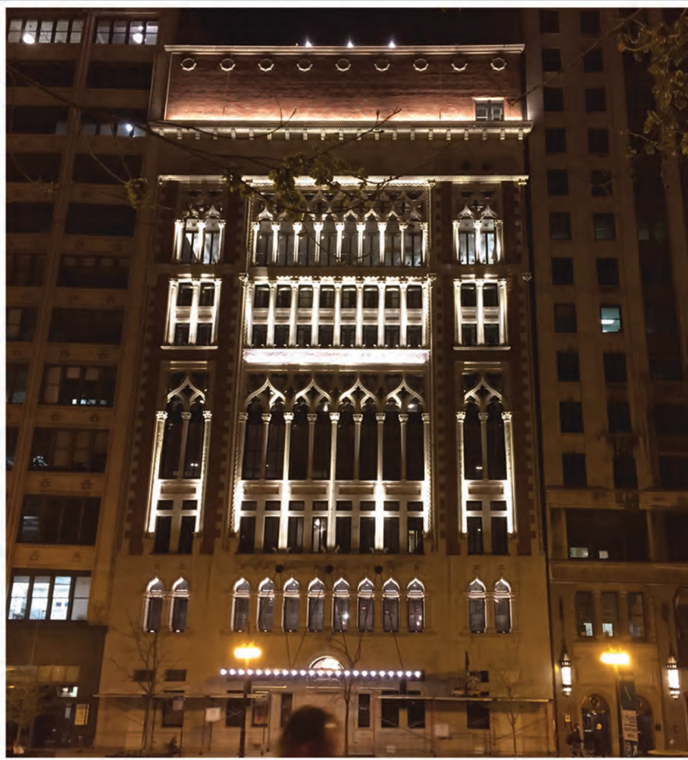
Block Electric recently completed a two-year renovation of the Chicago Athletic Association Hotel, which is located at 12 S. Michigan Avenue in the heart of downtown Chicago.
